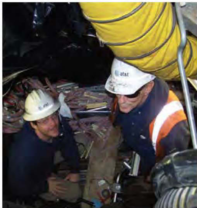
Tim Stacy and Terry Saunders are hard at work in a manhole splicing a cable on Route 30 in Frankfort.
